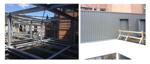
**Fig. 5.** Boiler plant new construction on terrace roof 4<sup>th</sup> floor: structure (left), finished (right)
