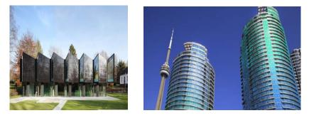
Figure 4. Thin film integrated in the facades of the buildings [4,5]
