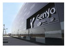
Figure 9. Photovoltaic panels with amorphous silicon glass modules with a semi-transparency degree of 20 [7]
