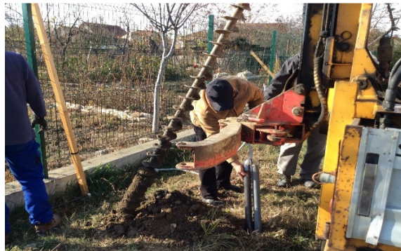
Fig. 6 Installation of the samples in the soil
