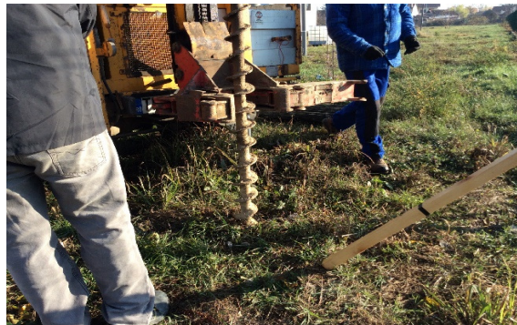
Fig. 2 Drilling operation in the ground
