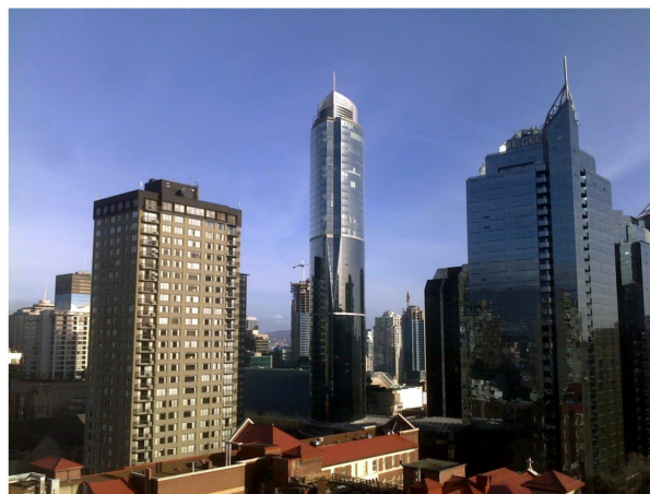
Fig. 3 One Wall Center, Vancouver, Canada
