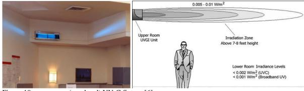
Figure 10 upper room (overhead) UV-C fixture [6]
