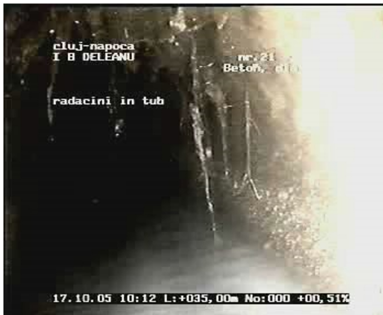
Fig. 2. Root intrusions in concrete sewer pipe [1], [2]. In this case the fault is in a more incipient state, the roots are long but not as branched out as in the previous image.
