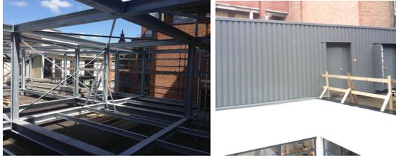
Fig. 5. Boiler plant new construction on terrace roof 4<sup>th</sup> floor: structure (left), finished (right)
