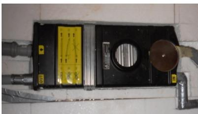
Fig. 11. Regenerative panel with stainless steel heat exchanger [6]
