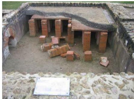
Figure 2. The first central “Roman” floor heating
