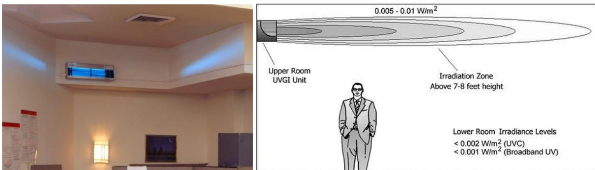
Figure 10 upper room (overhead) UV-C fixture [6]
