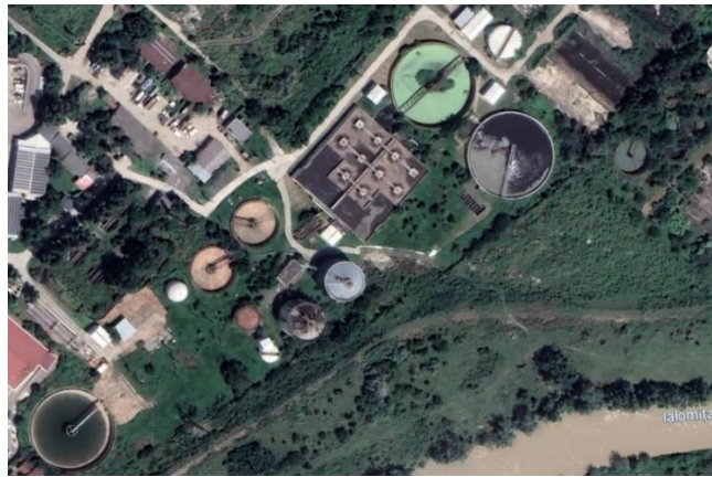
Figure 3 – Slobozia WWTP (Google Earth)
