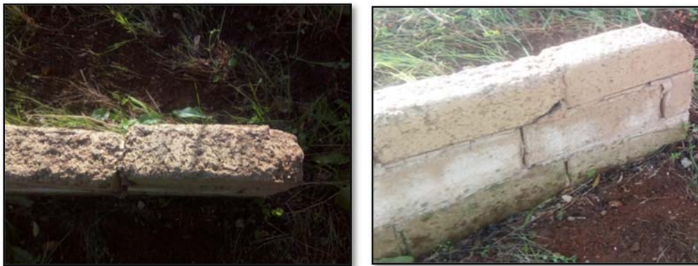
Figure 14: Wall condition stabilized by 10% lime (November 2020).
