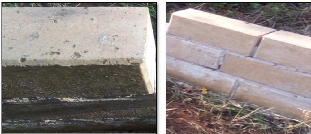
Figure 15: Wall condition stabilized with 8% cement (November 2020).
