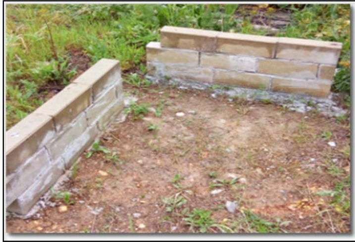
Figure 8: Walls built and exposed - February 2019.
