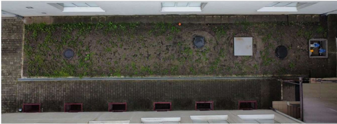
Fig. 4. Aerial view of the completed AmZEB pilot rainwater-harvesting system. Reproduced from Deac et al., Water 2026, 18, 731, CC BY 4.0.
