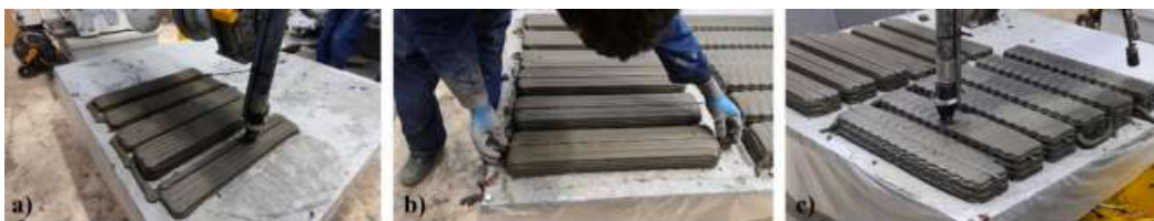
Fig 7 3D printed concrete beams process: a) printing of bed-surface layers b) placement of steel rebars c) printing of encasement layers. [9]
