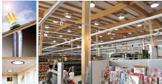
Fig. 9. Daylight guidance systems using light-pipes (source: Monodraught).
