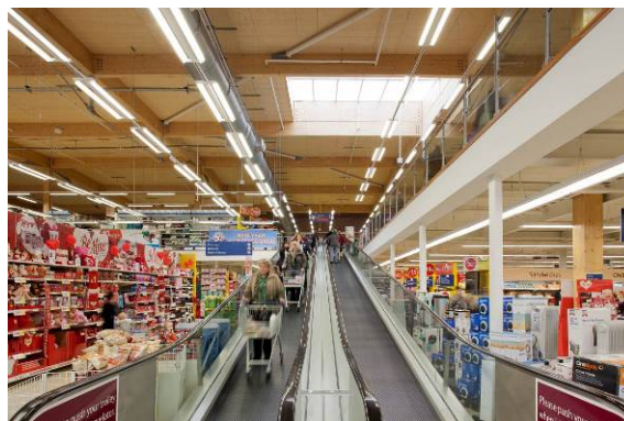
Fig. 11. Daylight-based, dimmable T5 fluorescent fittings with adjustable reflectors and louvres producing the right light output at the level of the merchandise (source: Whitecroft Lighting).
