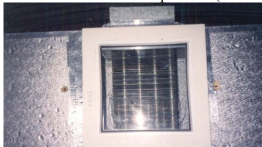
Photo 1. Finned air-cooler inside the air loop – plan view
