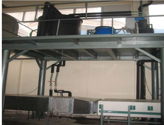
Photo1. Experimental stand showing the ice-slurry generation system on top, part of the air loop, containing the fan coil inside its lower branch and the connection tubes
