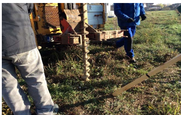
Fig. 2 Drilling operation in the ground
