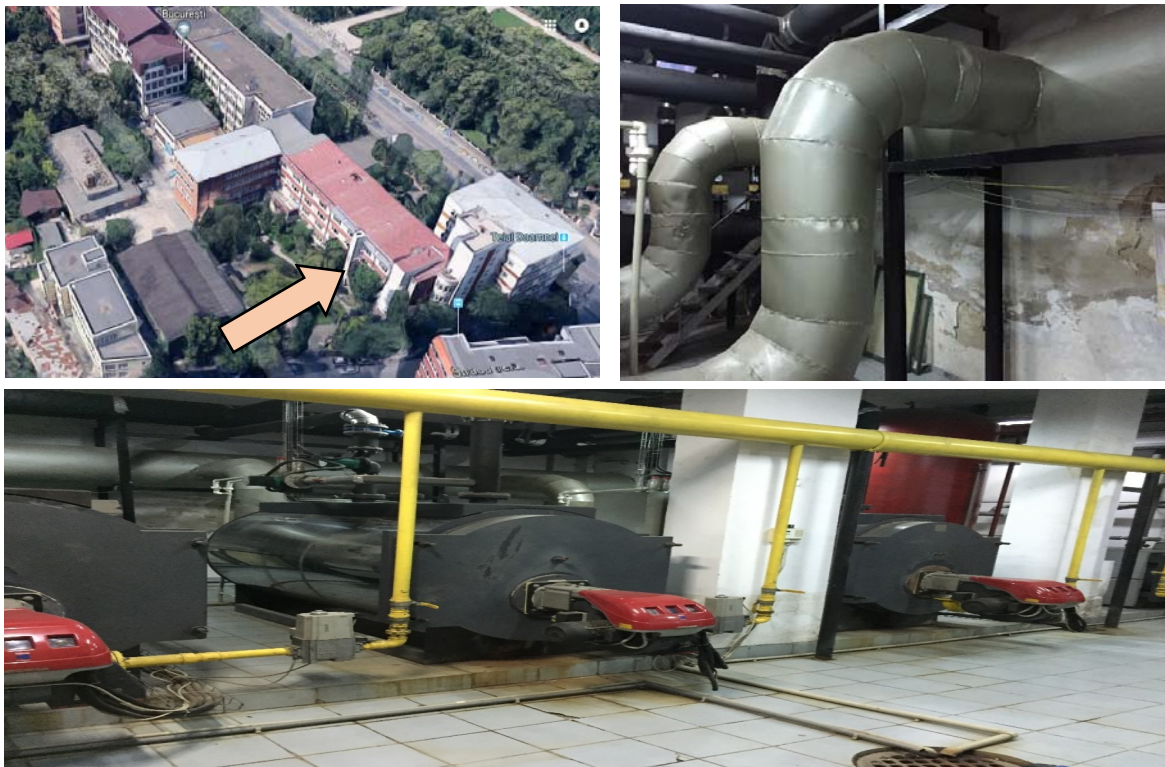
Fig.1 - Thermal plant. a) Boiler plant location b) Photo inside the thermal plant, c) Noise protection solution for the chimney
