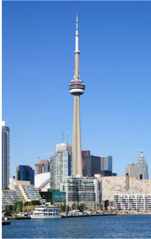
Fig. 2 CN Tower, Toronto Canada
