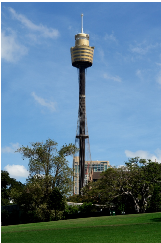
Fig. 1 Centerpoint Tower, Sydney Australia
