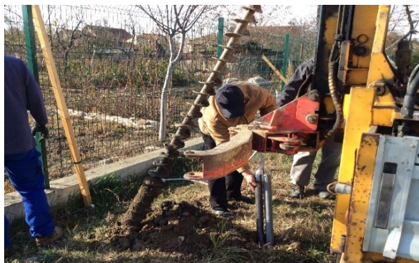
Fig. 6 Installation of the samples in the soil
