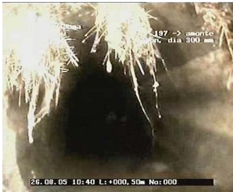
Fig. 1. Root intrusions in concrete sewer pipe [1], [2]. The roots are starting to branch already.
