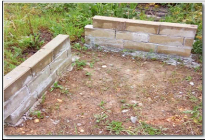
Figure 8: Walls built and exposed - February 2019.
