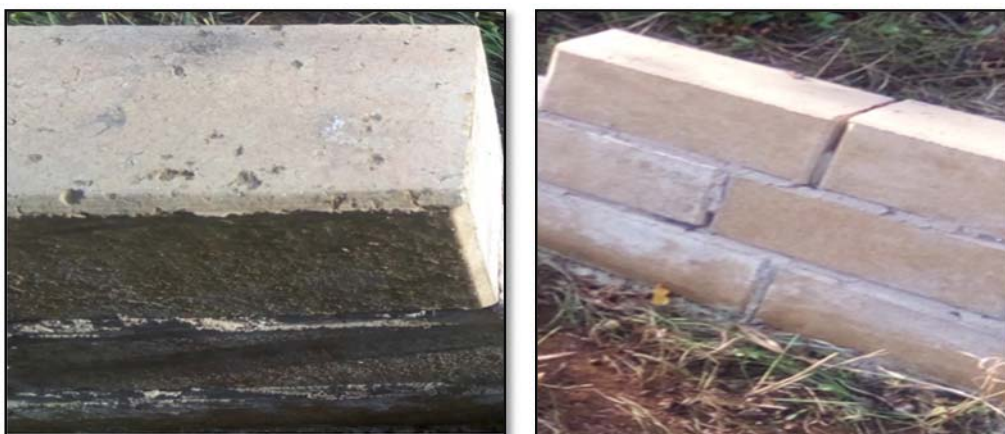
Figure 15: Wall condition stabilized with 8% cement (November 2020).
