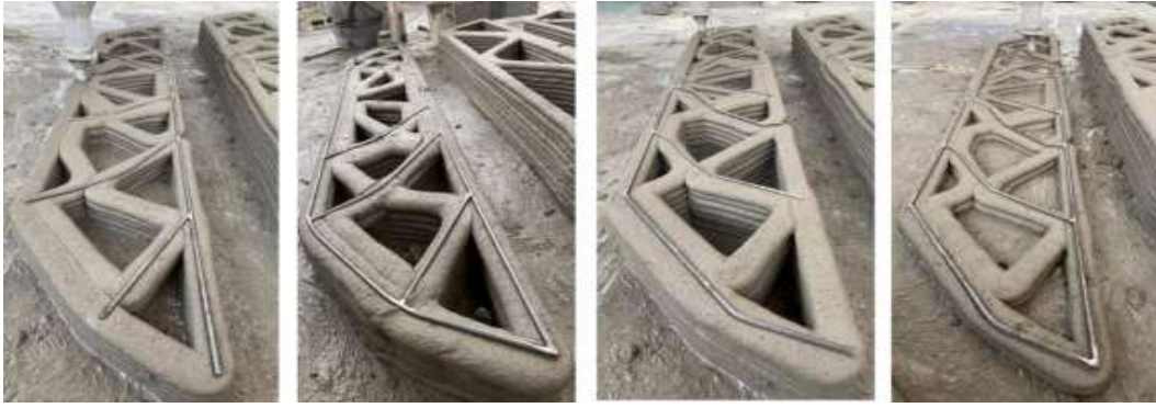
Fig 10 Reinforcement placement for different configurations. [10]
