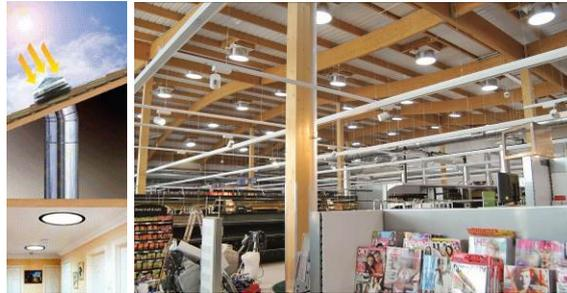
Fig. 9. Daylight guidance systems using light-pipes (source: Monodraught).
